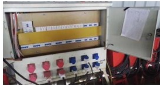
防砸、防雨挂牌上锁专人负责的二级箱 Anti - collision, anti - rain listing on the lock special person responsible for the secondary box
