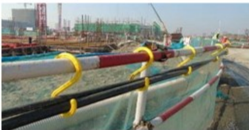
The cable is attached 电缆线系挂
